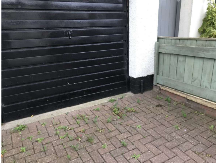
7.3. Gas pipe location to front right corner of property
