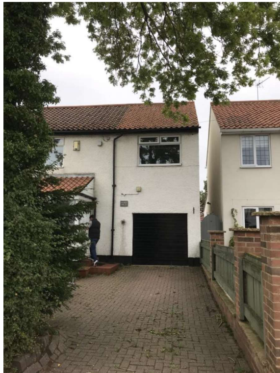
7.2. Partial front elevation and driveway
